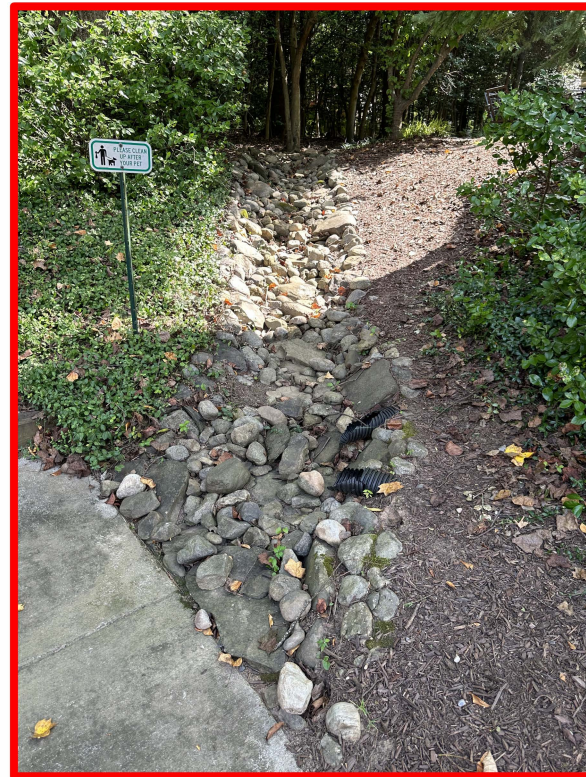
IMG_0536.jpg Channel 14 4' avg. width, 3-16" avg. stone size
