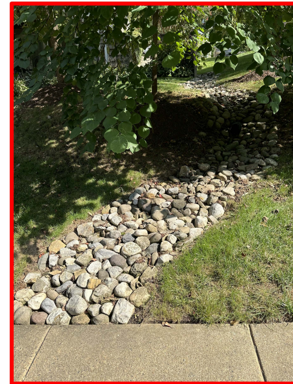
IMG_0538.jpg Channel 13 3' width, 5-6" stones
