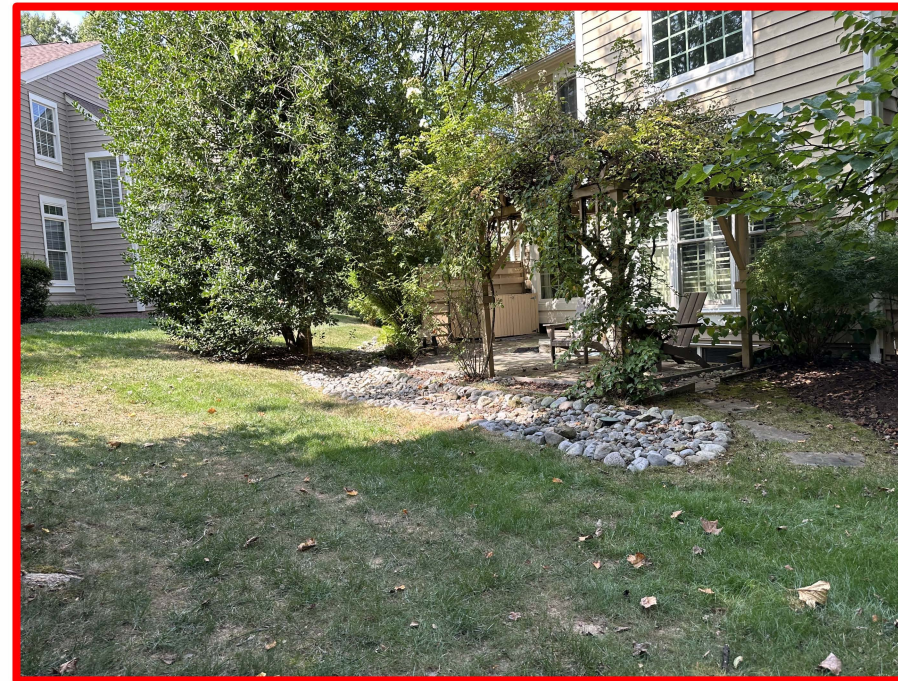
IMG_0529.jpg Channel 8 4' avg. width, 2-5" avg. stone size
