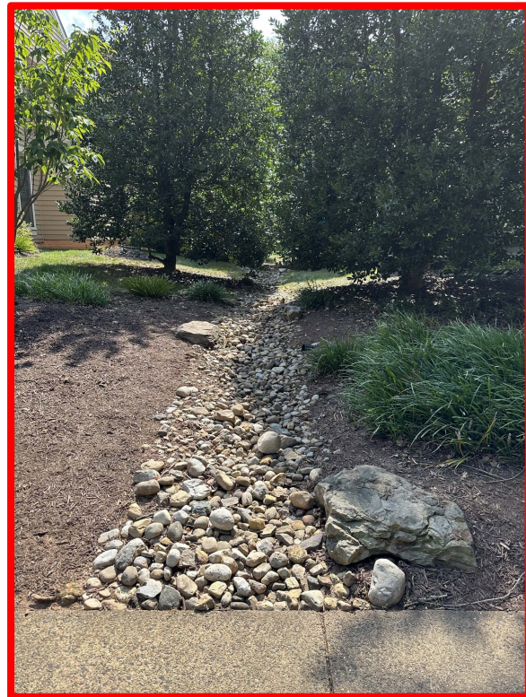
IMG_0526.jpg Channel 9 4' avg. width, 2-5" avg. stone size
