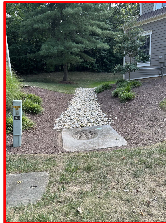
IMG_0537.jpg Channel 4 5' avg. width, 2-5" avg. stone size
